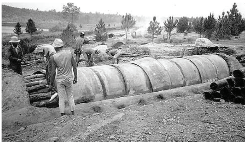
Figure 8: A semi-permanent low-cost “Subri-fosse” type metal kiln in Madagascar designed to carbonize off-cuts from sawmilling
