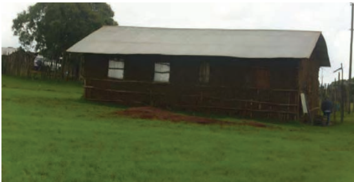
Plate 2: FTC in Weheni Durbete Kebele
