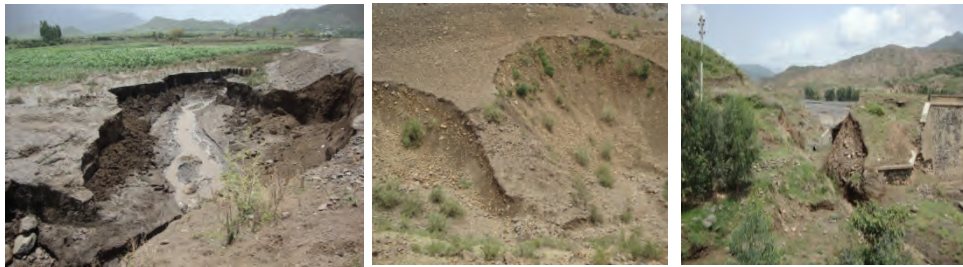
Plate 4. Flooding and soil erosion problems in Raya Azebo (above) and Meket (Below)
